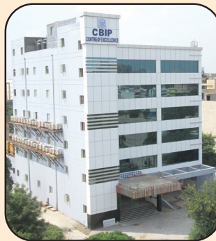
CBIP Centre of Excellence at Gurugram (2013 onwards) Sector 32, Plot No. 21
